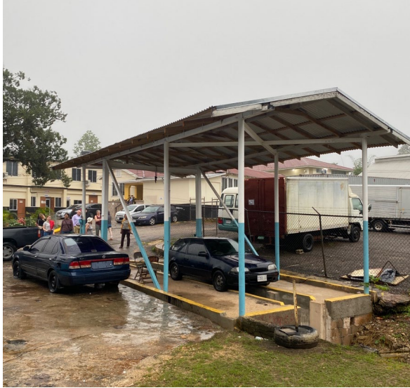
The auto repair pit with a new roof and repairs to the structure
