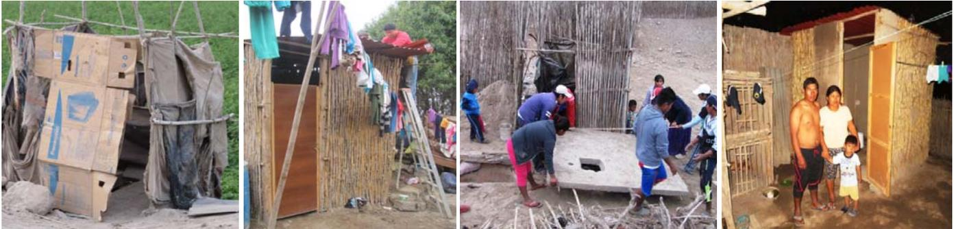
For this reason, a project was developed to assist Pachacutec community to build and use an improved system of waste disposal, which is hygienic and safe. An eco-toilet is a hygienic, waterless-composting human waste disposal system, which is being used in many South American communities that do not have a sewage system. This odourless system is very efficient, and human waste can be properly composted to make it suitable for growing crops.
