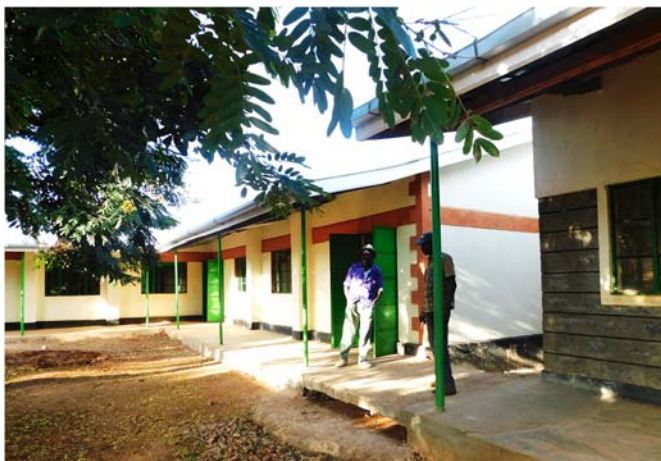
Outside of new buildings
